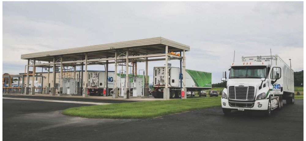
XNG, a Massachusetts-based logistics and transportation company, was granted a 10-year lease for a 4.3 acre parcel in the West Park area of Satsop Business Park where they will construct a natural gas filling station, similar to the one pictured above, to serve various industrial customers, currently without access to natural gas, with compressed natural gas delivered via all-composite trailers. Photo credit: Xpress Natural Gas, LLC
